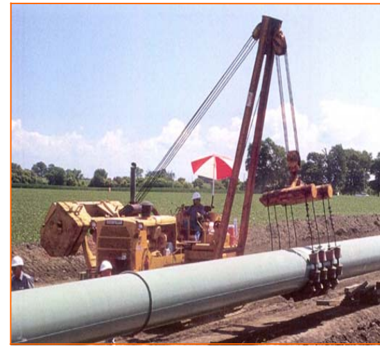
Pipeline Structures All types of Cross country pipelines for oil, gas and water.
