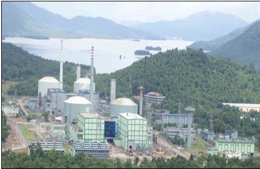
Kaiga unit 3 & 4 – 450MWe, Karnataka
