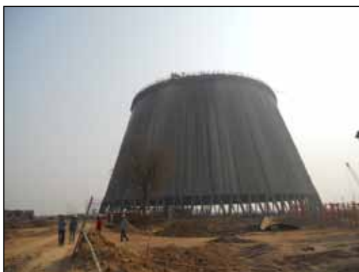
◀ NDCT - 1 Shell in Progress at GMR Energy, Raipur
