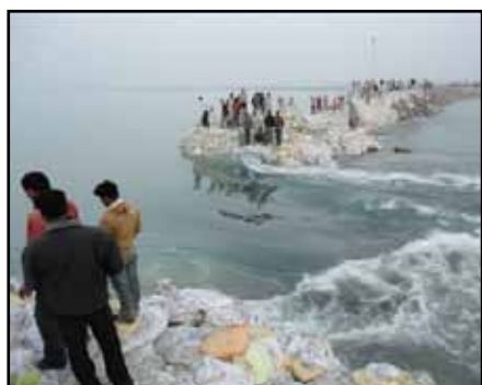
Photo 2 : 12 meter blockage; level difference three meters.
