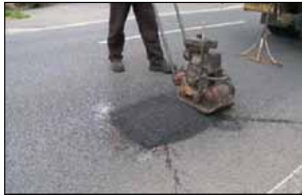
Photo 4: Pothole Repair by Semi Permanent
