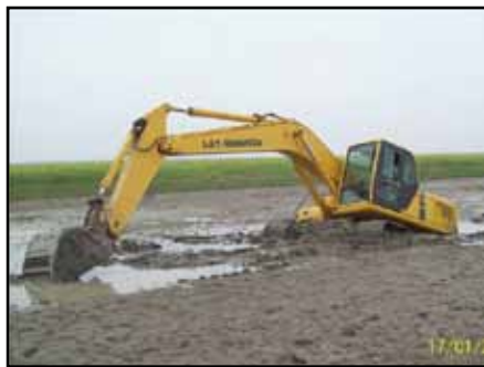
Photo 1 : Condition of excavators for making Pilot Channel
