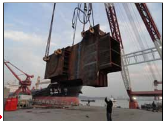
Signature Bridge : Pylon Base (360 T) - Mock assembly in China ▶
