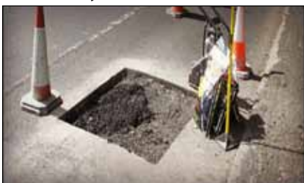
Photo 3: Cutting Pothole to Proper shape
