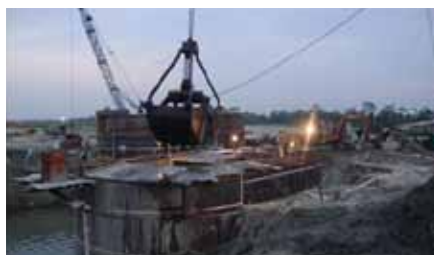
Fig-28: Grabbing inside the Caisson for Floating into the water
