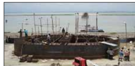
Fig 38: Cutting edge modules erected
