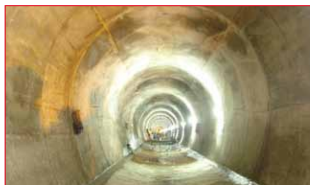
Submarine tunnel under the sea for sea water intake at Kalpakkam
