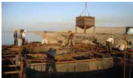
Fig-32: Concreting by using Crane & Bucket
