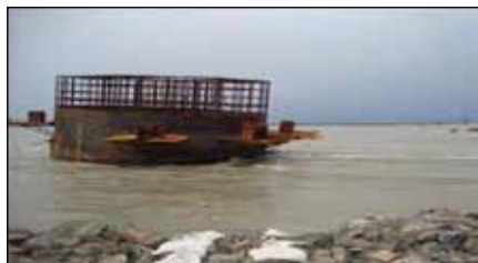
Fig-6: P2 Caisson drifted 130m downstream
