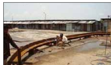
Fig-14: Placement of the bent angle
