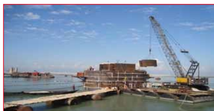
Fig-31: Erection of Further Modules at Location
