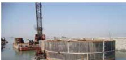
Fig-4: P2/ P3 caissons shifted to actual location
