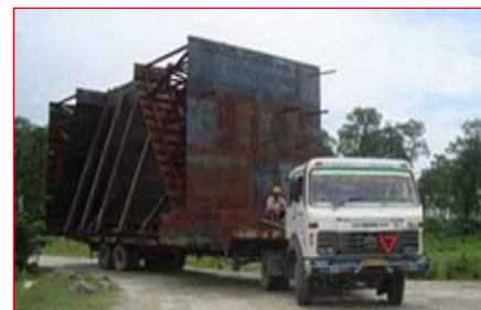
Fig-24: Shifting of Pre-Fabricated Caisson Module
