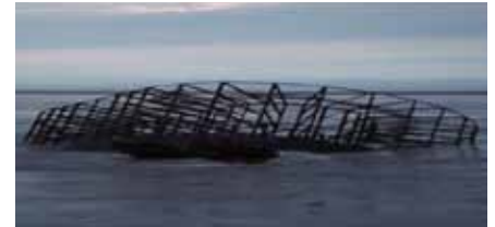
Fig-8: P3 caisson submerged in river
