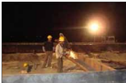
Fig-16: Fixing the diaphragm angle
