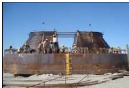
Fig 39: Cutting edge erection completed
