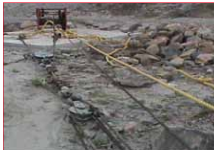
Fig-12: Revised winch arrangement from ground anchor
