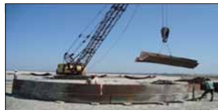
Fig 35: Erection of Fabricated Modules of Cutting Edge
