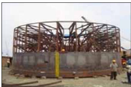
Fig-18: Fixing of inner & outer skin plates & Hoop angles
