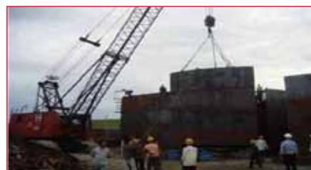
Fig-23: Lifting of the Curb (5.1m) portion
