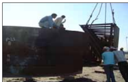
Fig 37: Erection of Cutting edge modules at location
