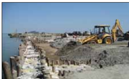
Fig-25: Coffor Dam for Launching of Caisson
