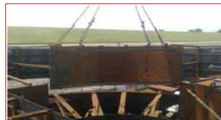
Fig-22: Lifting of Cut Piece of Modules
