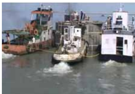
Fig-29: Caisson being towed to location
