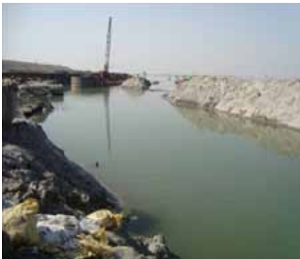
Fig-3: Dredging of River for Shifting of Caisson
