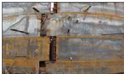
Fig-21: Cutting of Caisson in Modules
