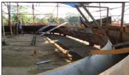
Fig 33: Cutting Edge Fabricated up to 1.0 mtr. height
