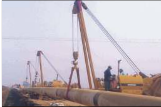
Paradip Haldia Pipeline
