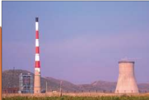
Bellary Cooling Tower & Chimney
