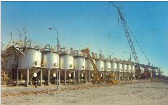
Dubai dasltn plant
