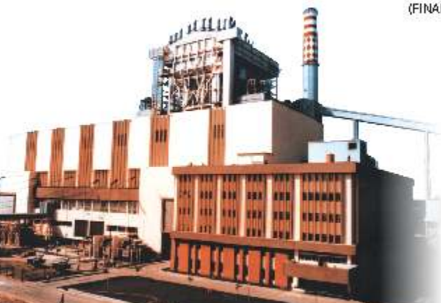
Tata Trombay Thermal Power station
