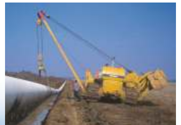
Paradip Haldia Pipeline
