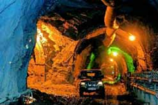
Farhadi Tunnel Work
