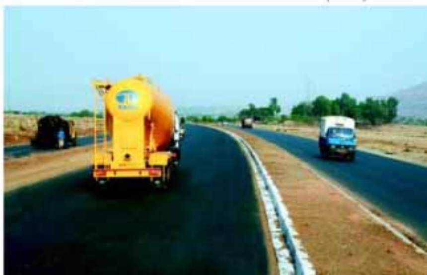
Mumbai Nashik Expressway Ltd.
