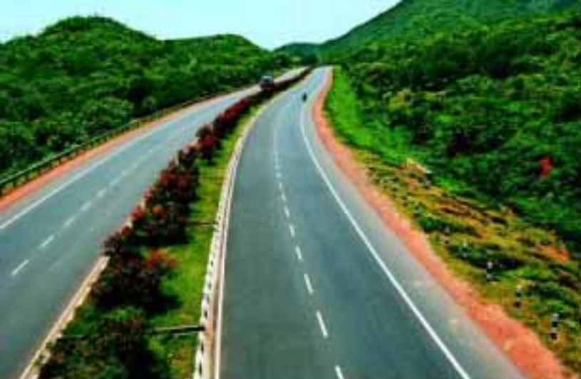
Rajahmundry Expressway Ltd.
