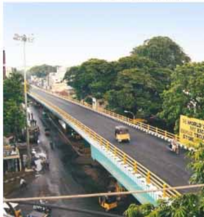
Westcott Road Flyover, Chennai
