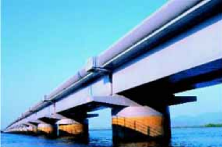
Vival Creek Bridge
