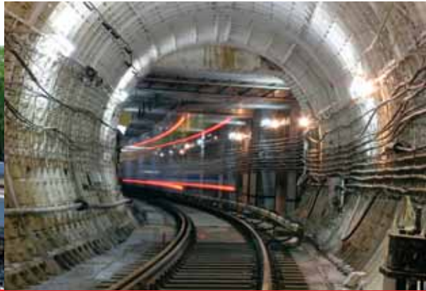
Chennai Metro Tunneling
