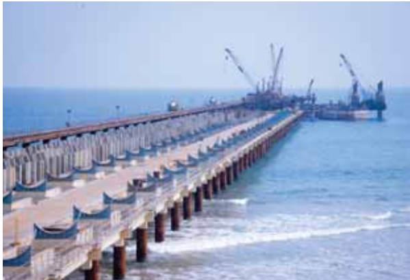
Sea Water Intake for Hinduja Power
