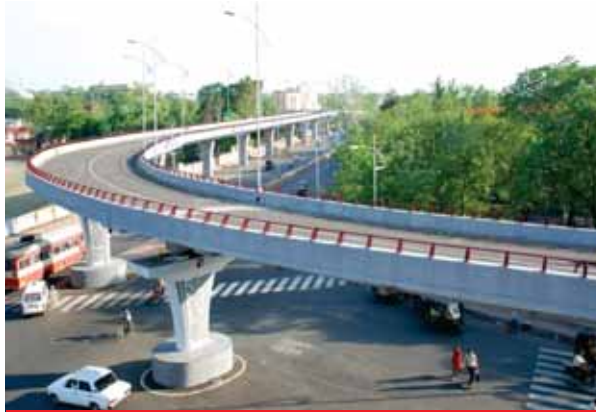
Panchvati Flyover, Amravati
