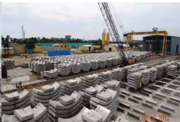
Chennai Metro Casting Yard
