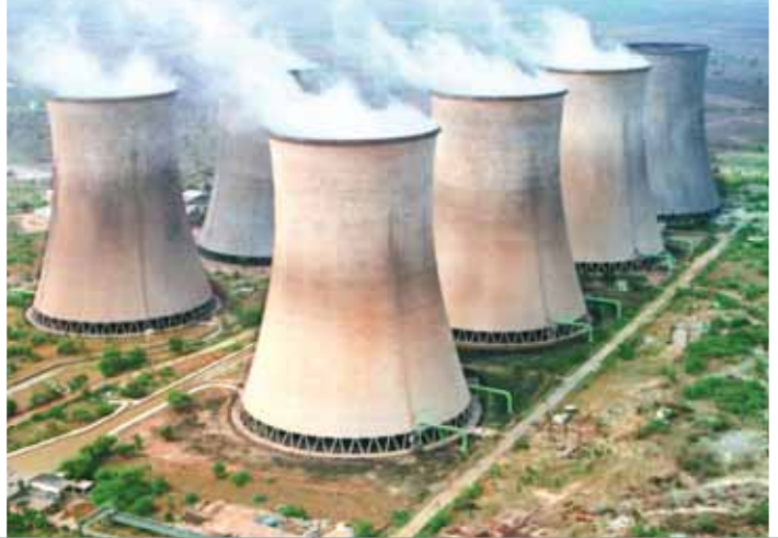
Thermal and Industrial Thermal Power Plant Steel Plants Cooling Towers and Chimney
